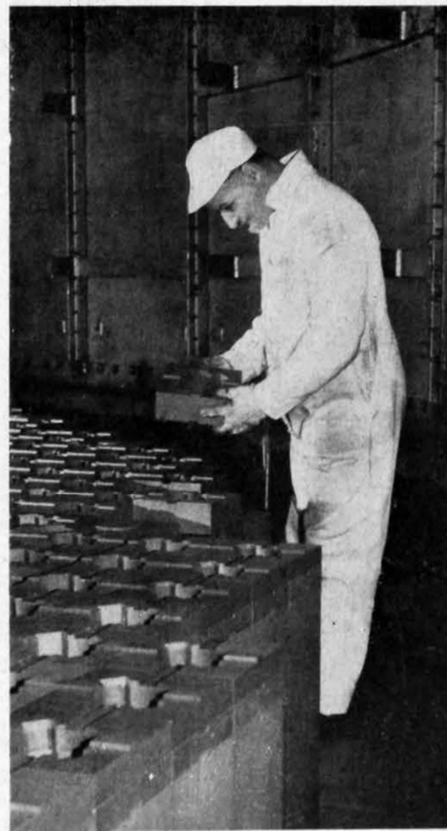
Fig. 2—The first layer of the graphite is nearly completed
