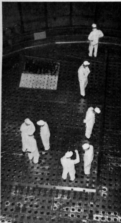
Fig. 1—4in thick steel support plate for graphite core. The straight edges define the first quadrant
