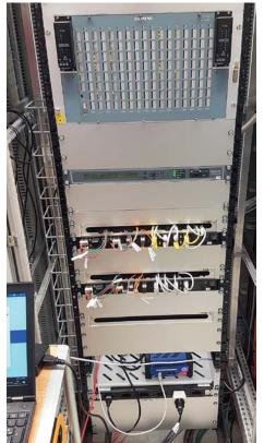
Figure 2 shows the installation using the mobile hardware platform MBX1 at the bottom of the picture. In this setup, all traffic of the "core" switch was mirrored to StationGuard.
