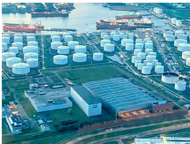
GPS Amsterdam Terminal, facility for storing and blending gasoline, oil, and bio fuels (Source: Wikipedia)
