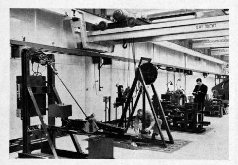
The new building also includes a fuel injection equipment bay and a temperature-controlled room for carburetter airbox testing; the continuous flow rig is seen ABOYE. The long-term stability of streamline metering orifices is valuable, as there is no positive displacement rig against which to calibrate them.
