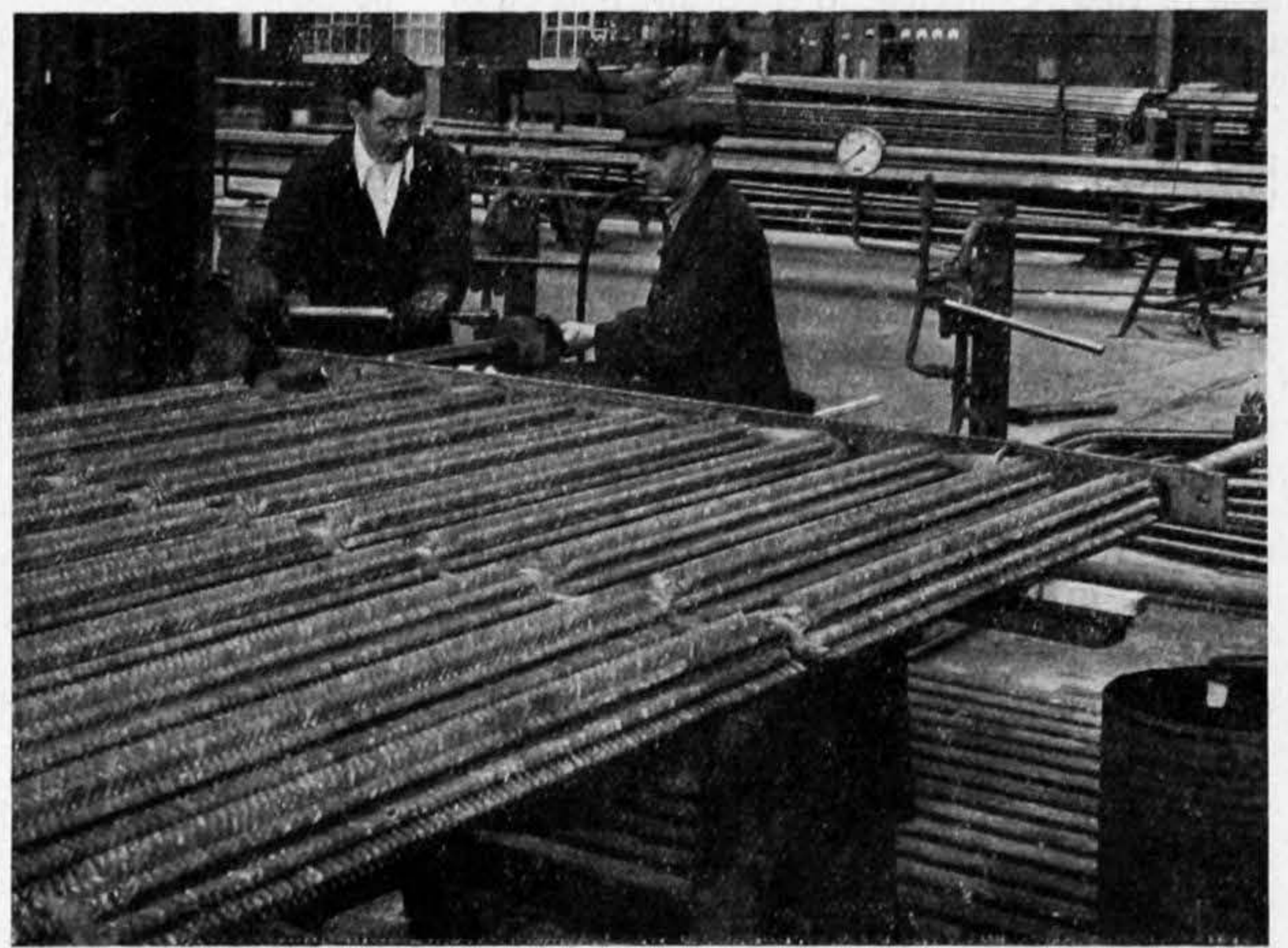
Figs. 4 and 5—(Left) the bottom of the reactor pressure vessel casing. Carbon dioxide for cooling the reactor core is pumped at 100 lb per square inch into the bottom of the pressure vessel through four inlet ducts, part of which can be seen. (Right) a heat exchanger section rigged for hydraulic testing. The surface area of about 30,000 square feet of the complete heat exchanger is made up of several million welded studs of aerofoil section
